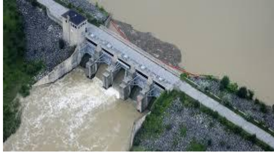
Fig.4 Dam Constructed for Flood Mitigation
