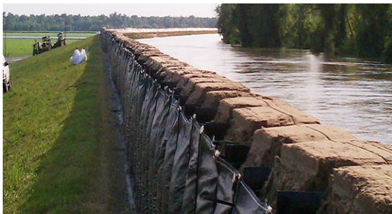
Fig.3 Levees for Flood Mitigation
